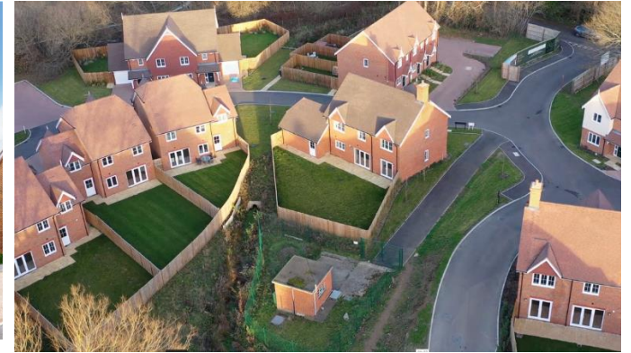
Photo 6: Weyburn Works, Elstead
